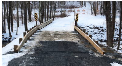
Poultney-Mettowee NRCD helped replace an undersized culvert with a sixty-foot bridge on the Mettowee River, restoring aquatic organism passage in one of the best trout streams in Vermont.
