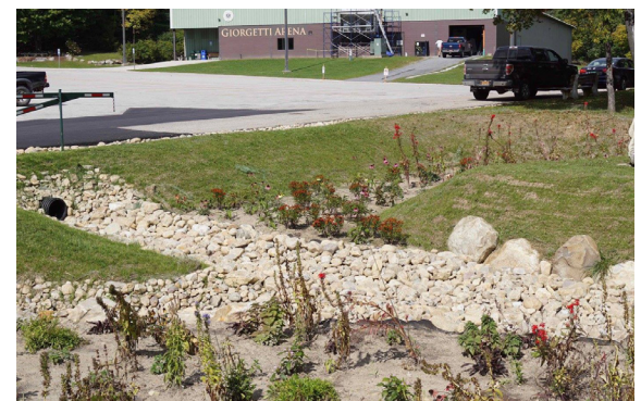
This Bioretention Basin at Giorgetti Park implemented by the Rutland NRCD reduces pollution and nutrient runoff, increases flood resiliency, prevents additional stream bank erosion, & helps protect water quality.
